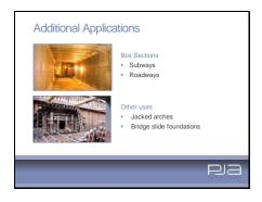
In addition to conventional conduits pipe jacking has a variety of specialist applications. These include box sections for subways and roadways, bridge foundations for bridge slides and also jacked arches.
