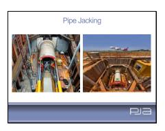
A range of machines are available, to suit varying ground conditions, to install pipes typically in the range 150 to 2,400 mm or greater if required. Lengths of up to a kilometre or more can be jacked depending on ground conditions and pipe diameter. Drives can be either in a straight line, to a radius or a series of radii. Concrete, Grp, clay and steel pipes can be jacked.
