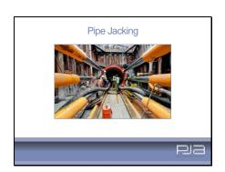
Pipe jacking is a tunnelling technique for the installation of pipes using powerful hydraulic jacks to drive purpose designed pipes through the ground at the same time as excavation is taking place at the face.
